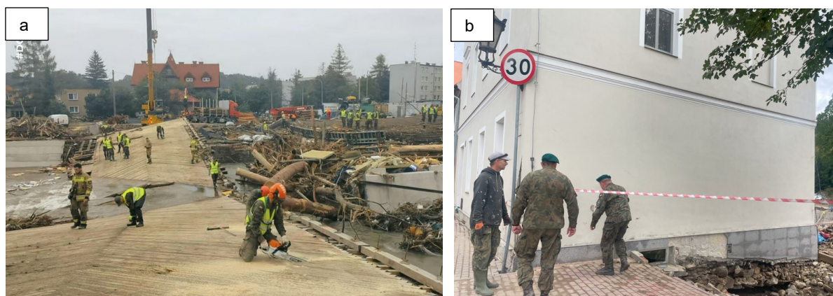
Fig. 1. Activities of Polish soldiers during the fight against the effects of the flood: a) removal of a damaged temporary bridge structure; b) assessment of the technical condition of a building damaged as a result of the flood
